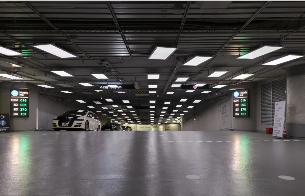
Functional light panels are arranged in pixelated arrangement to create an unexpected ceiling feature.
