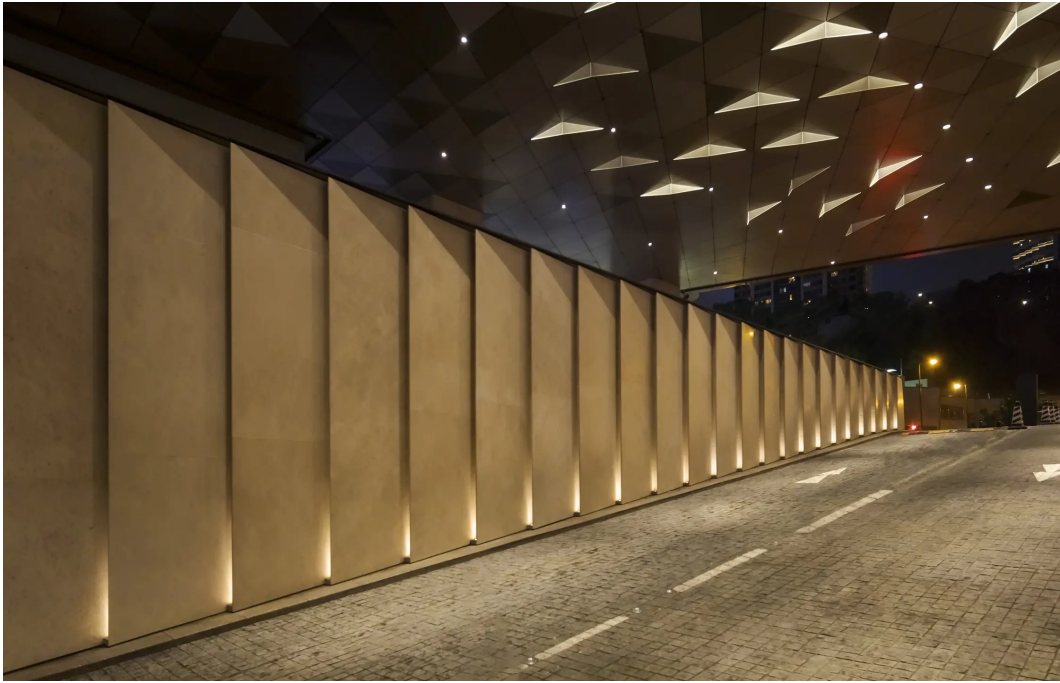
Rhythmic wall mounted light features at the entrance ramp provide the required light levels by day and by night.
